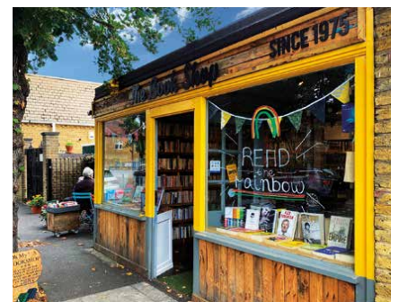
The refurbished shop front ▲
